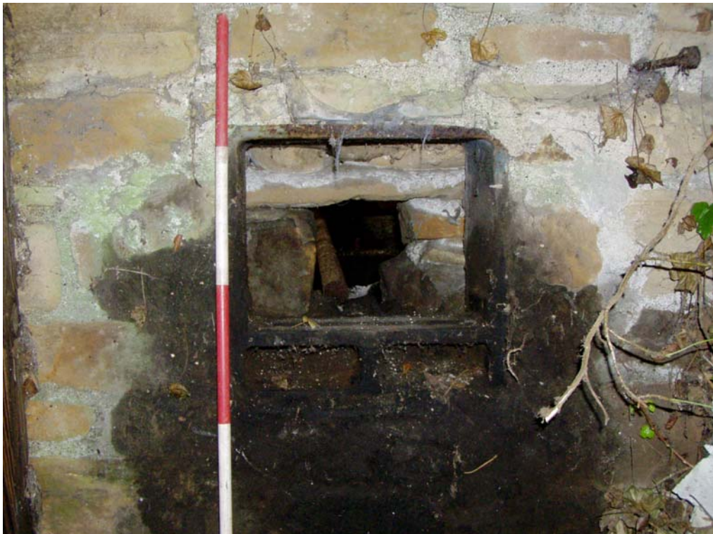
Plate 8: Bearing box in south elevation
