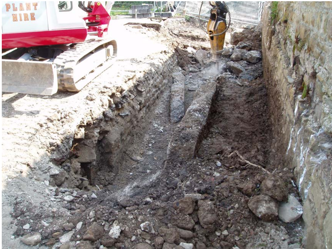
Plate 16: The concrete and stone-lined channel ( 106 and 109 ) during excavation
