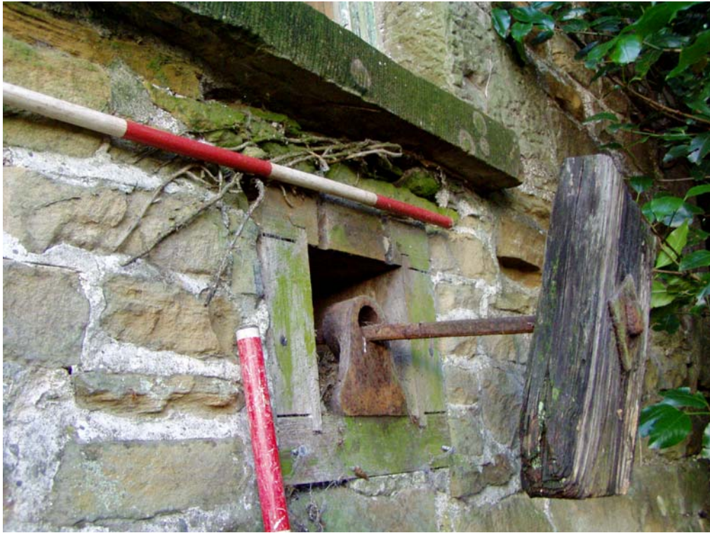
Plate 7: Bearing box beneath window on east elevation
