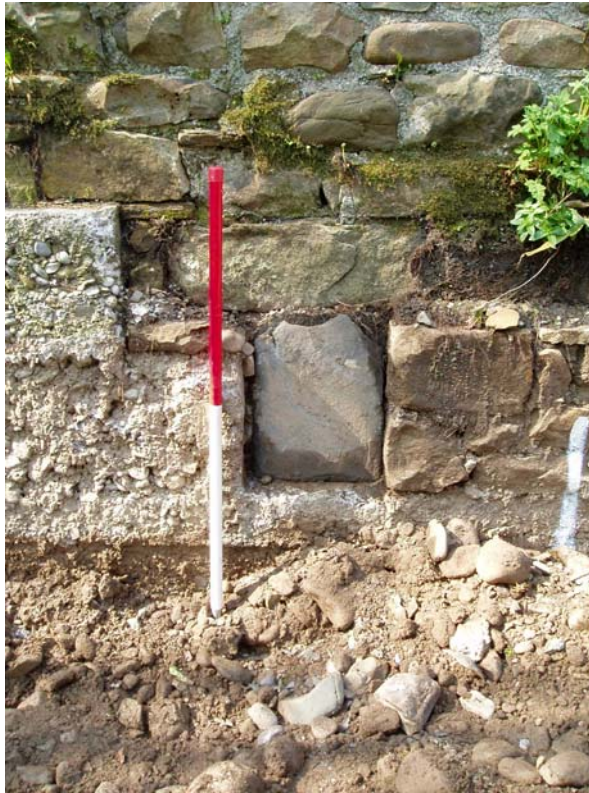
Plate 14: Blocked aperture in the east elevation of the mill, uncovered during the watching brief
